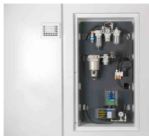
Through centralized management of pneumatic solenoid and lubricant pump, it made the daily maintenance easy.
